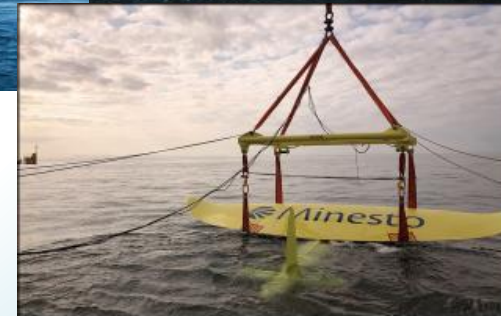
Figure 3.5. Minesto's Deep Green 0.5 MW tidal kite being deployed at Holyhead Deep, in Anglesey, Wales. (Photo courtesy of Minesto)
